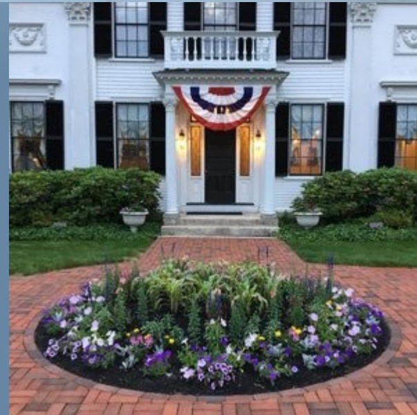
Left-One story porch with full Corinthian entablature topped by flat roof with balustrade
